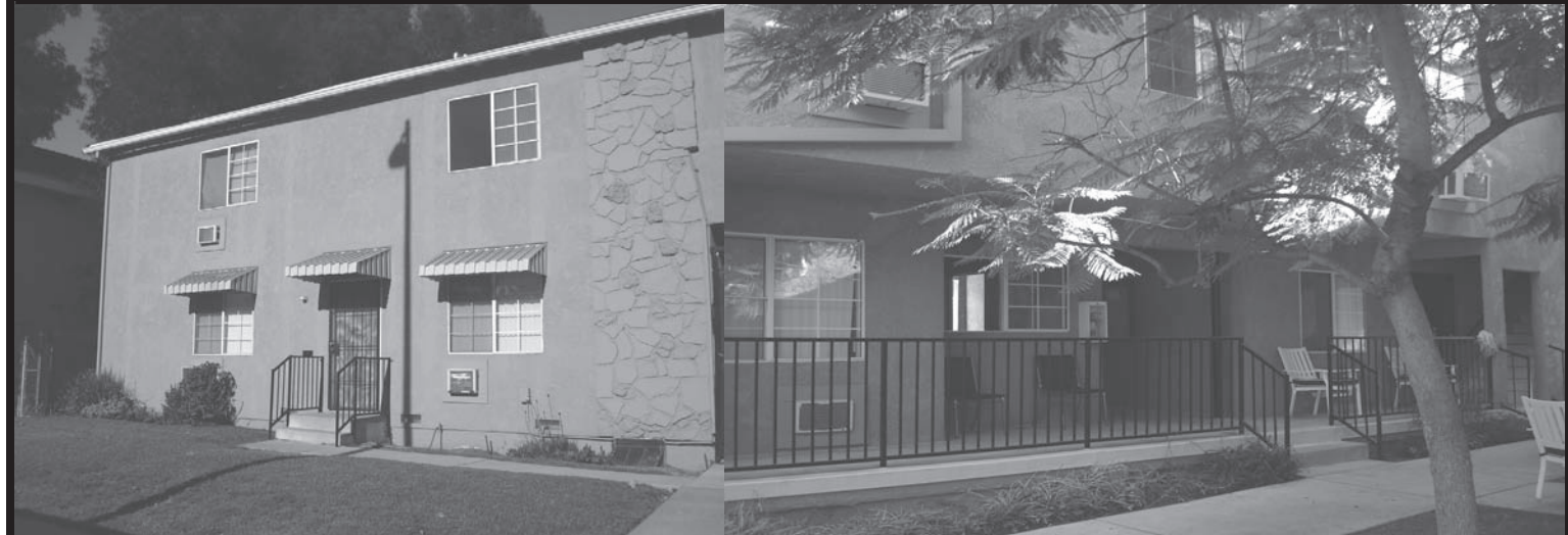
TOP LEFT: The building gets ready for its facelift! TOP RIGHT: Volunteers from Bel Air Presbyterian are on hand to help! ABOVE LEFT: The new front of the Shared Living Community. ABOVE RIGHT: The new courtyard is a pleasant place to hang out!
